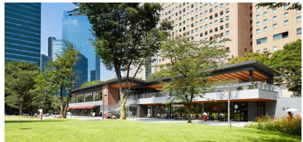
Photo ©2020 Nacasa & Partners Inc.
